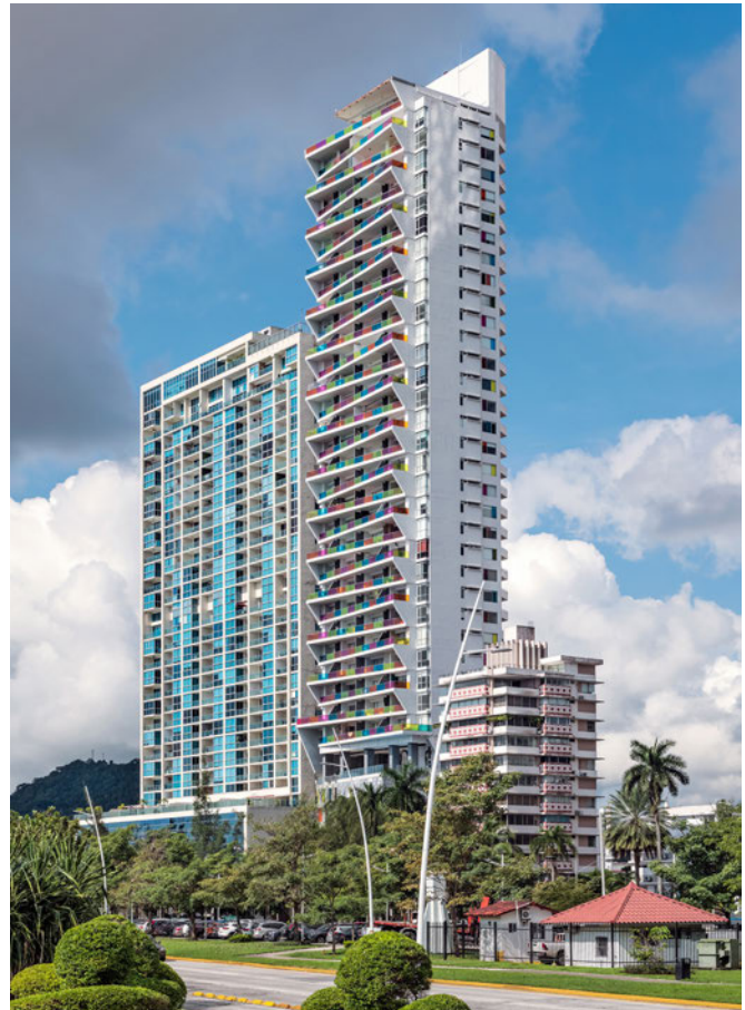
Tall residential buildings in Avenida Balboa
